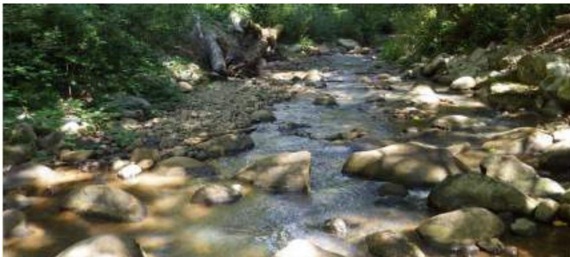
Figure 4-2. Example of a typical constructed roughened channel grade control using oversized coarse materials.
