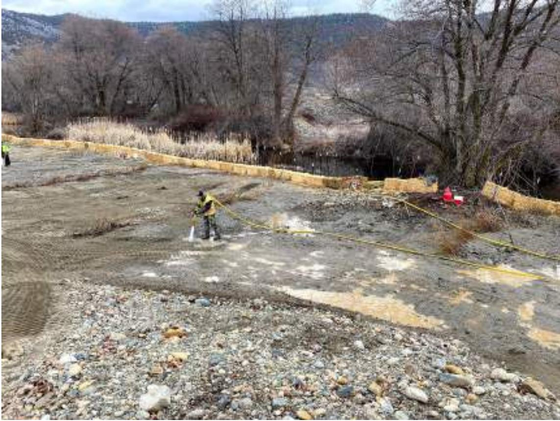
Figure 4-3. Typical application of fine substrate supplementation to treat coarse substrate void space and reduce the potential for stream flow loss.
