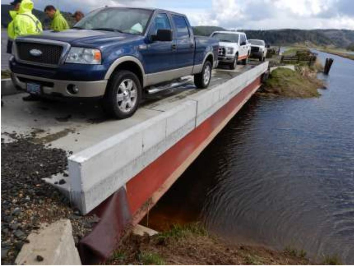
Figure 4-5. Example pre-cast concrete slab on steel girder bridge.
