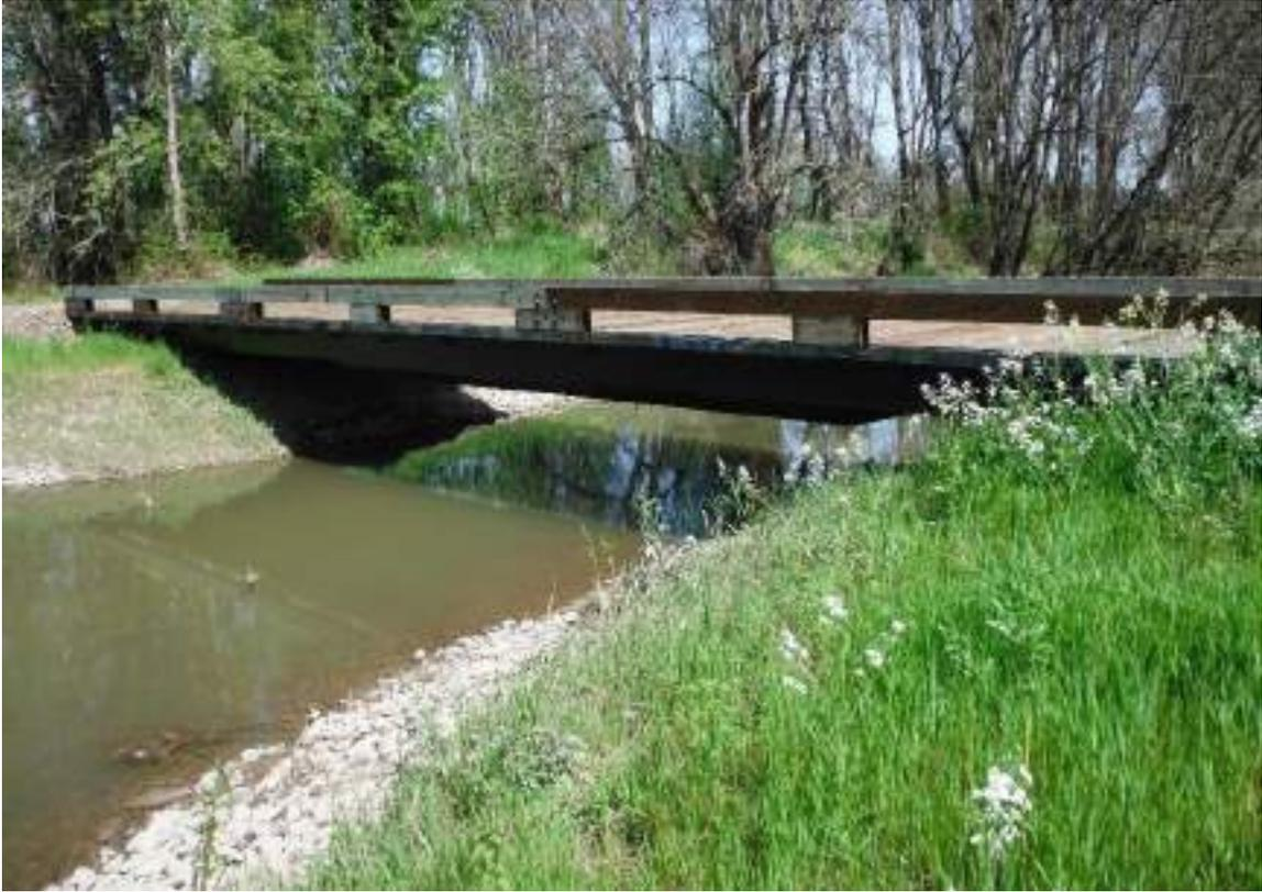
Figure 4-4. Example wood decked repurposed railroad flat car bridge.
