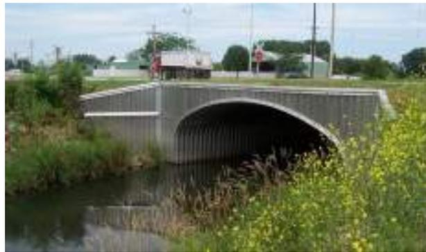
Figure 4-6. Example aluminum culvert.
