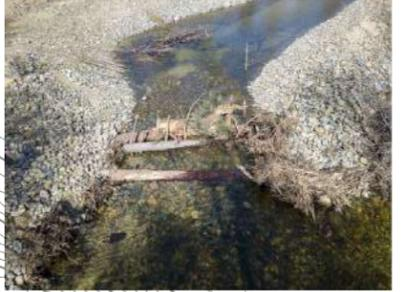
INSTALLED TWO LOGS AND A ROOTWAD
