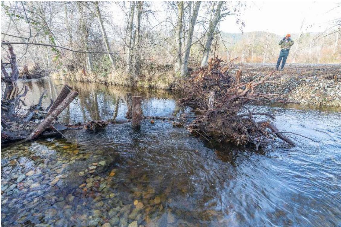
*Photograph 8. Channel Spanning Wood Structure*
