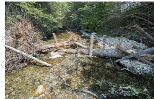
CHANNEL SPANNING WOOD STRUCTURE AND GRAVEL AUGMENTATION
