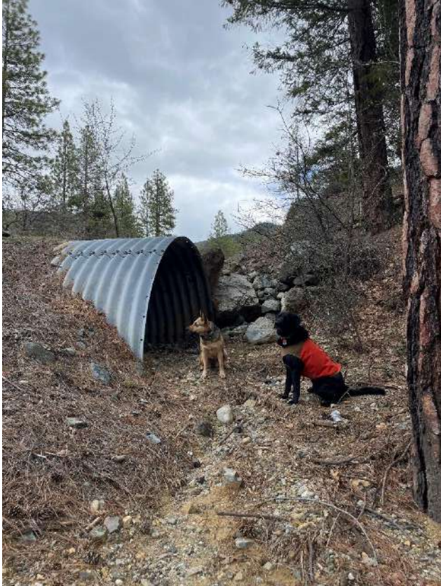
Photo 2.17: Beginning of EFG 24. Inboard ditch flows past culvert. EFG24a; April 5, 2024.
