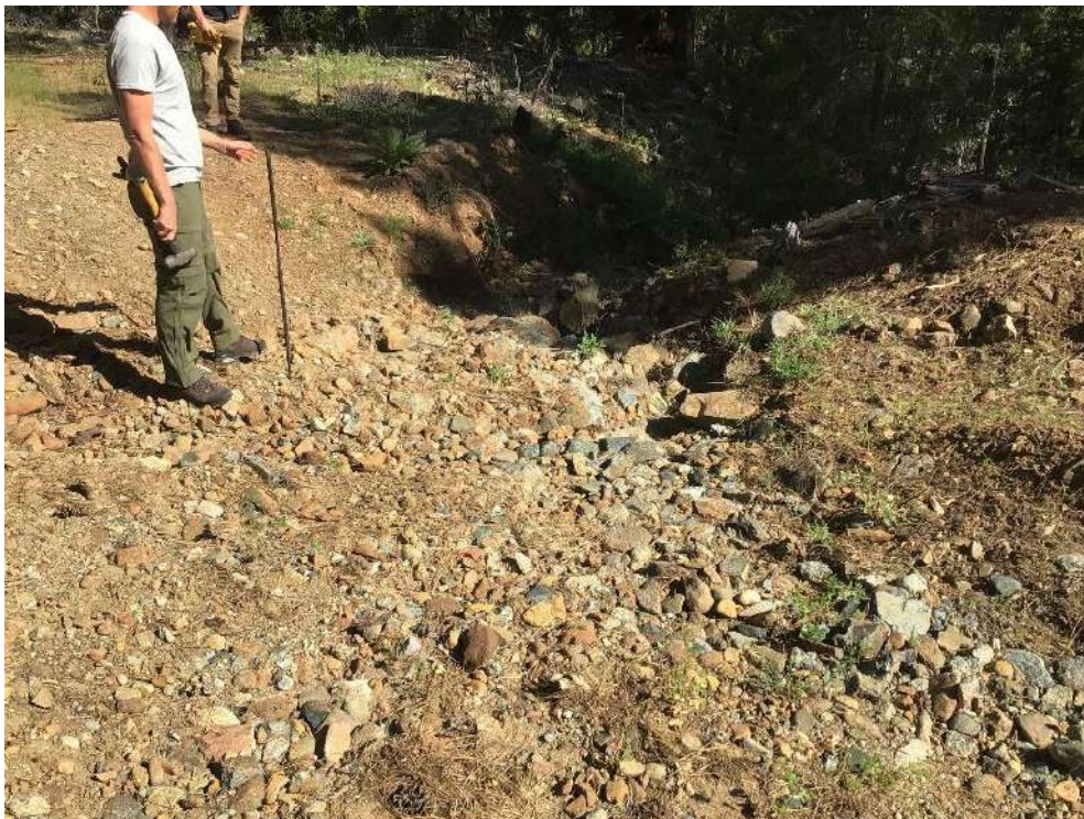
Photo 2.48: Gully Complex 5 road crossing. EFR6. May 23, 2023.
