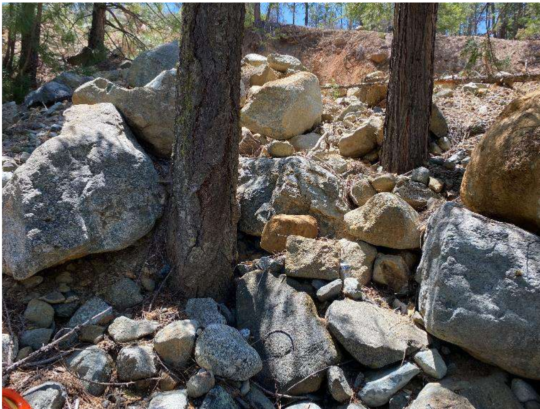
Photo 2.15: Below Highway 3 outboard ditch. EFG6.5.2c; June 2, 2023.
