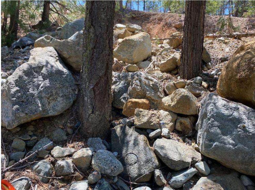
Photo 2.45: Below Highway 3 outboard ditch. EFG6.5.2c. June 2, 2023.
