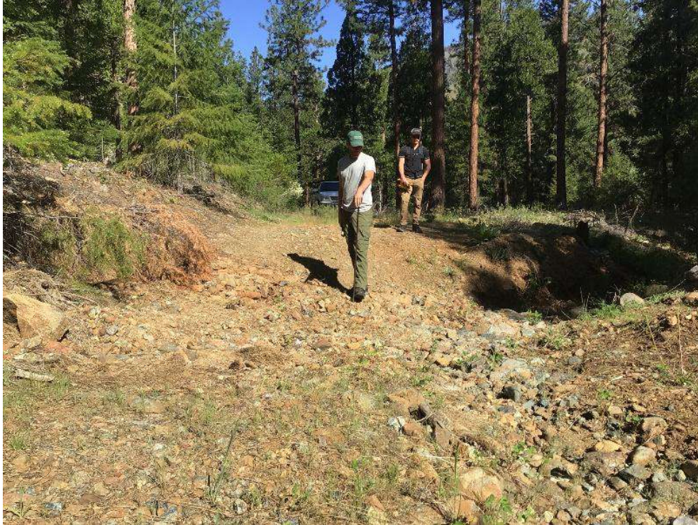
Photo 2.47: Gully Complex 5 road crossing. EFR6. May 23, 2023.
