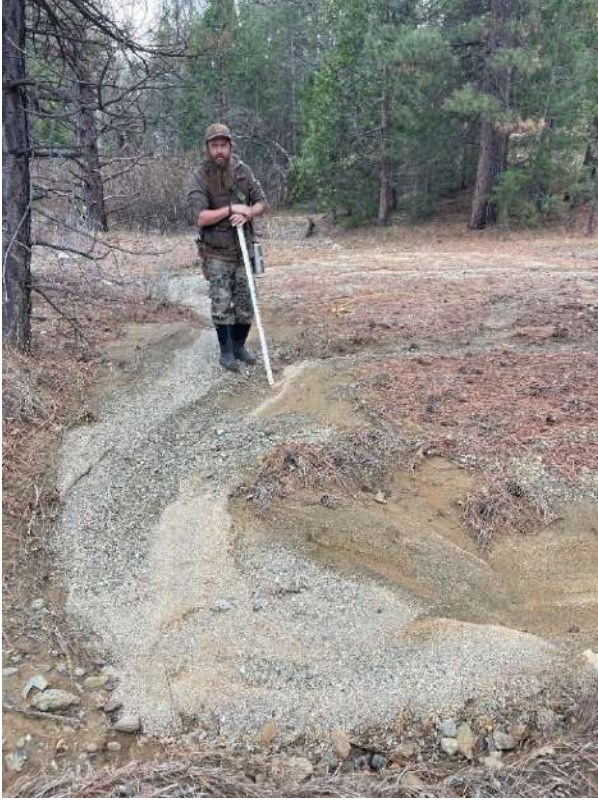
Photo 2.13: Sediment deposited by Gully Complex 2. EFG2f. January 19, 2024.
