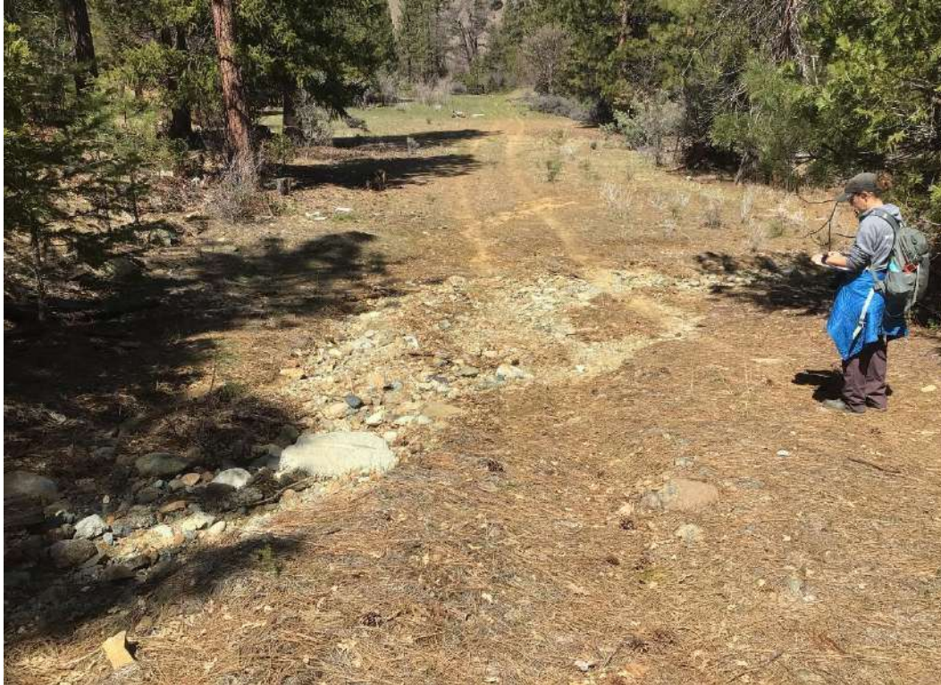
Photo 2.3: Example of extreme erosion point, EFR13.1; April 13, 2023.
