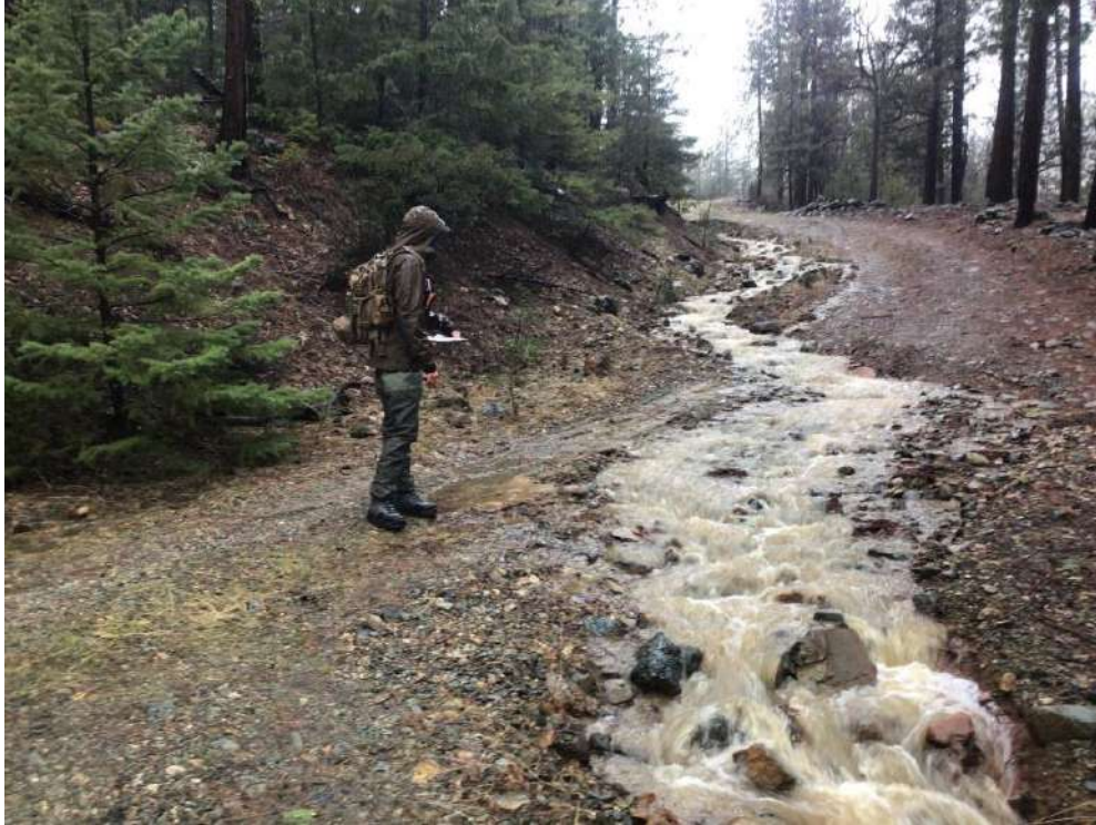
Photo 2.5: Water during runoff event crossing road, looking upslope. EFR2. January 13, 2023.
