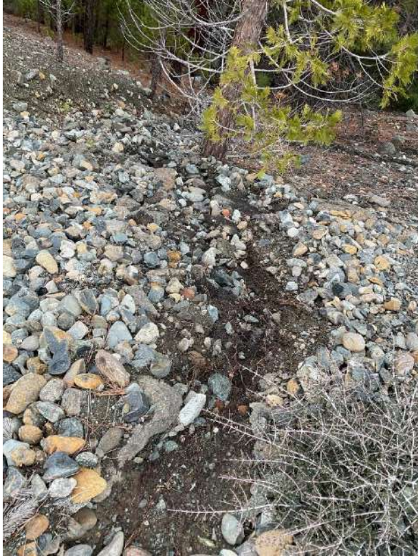
Photo 2.36: Discharge from outboard ditch erodes fill at the top of Gully Complex 12. January 18, 2024.
