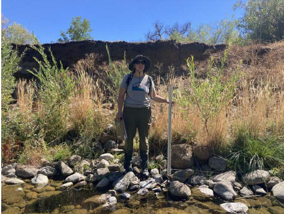
Cutbank at RKM 4.2 - illustrating riparian vegetation at toe of eroding bank
