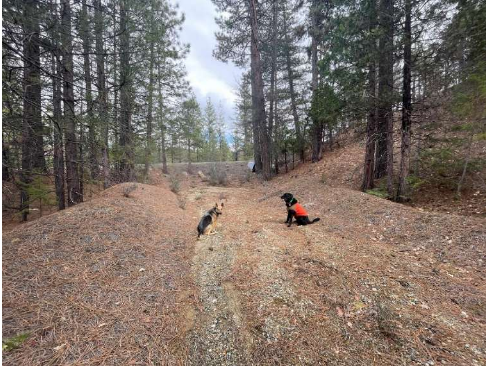
Photo 2.52: EFG 24 downstream of bypassed culvert. April 5, 2024.
