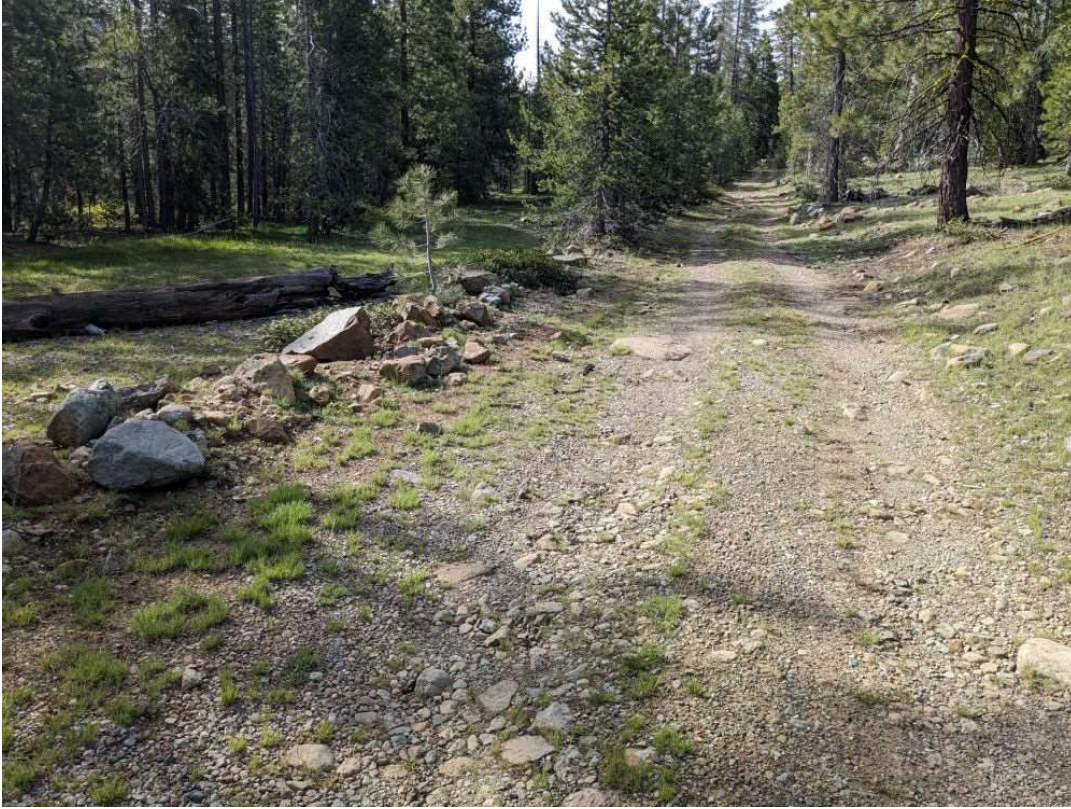
Figure 4-47. Looking south and upslope along road segment CM-17. An outboard berm is visible to the left which concentrates runoff on the road surface.
