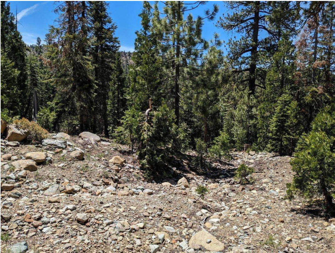
Figure 4-44. Looking downslope from STX-2, where a small watercourse has been diverted down the CM-5 road segment, resulting in surface erosion.
